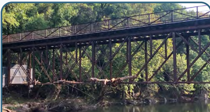
DEMA helped coordinate federal funding for the Bancroft Bridge Replacement Project in Wilmington.
